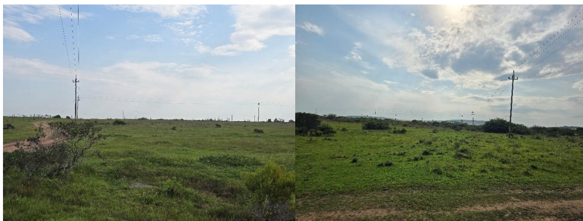
Figure 45: Existing powerlines within the Project site
